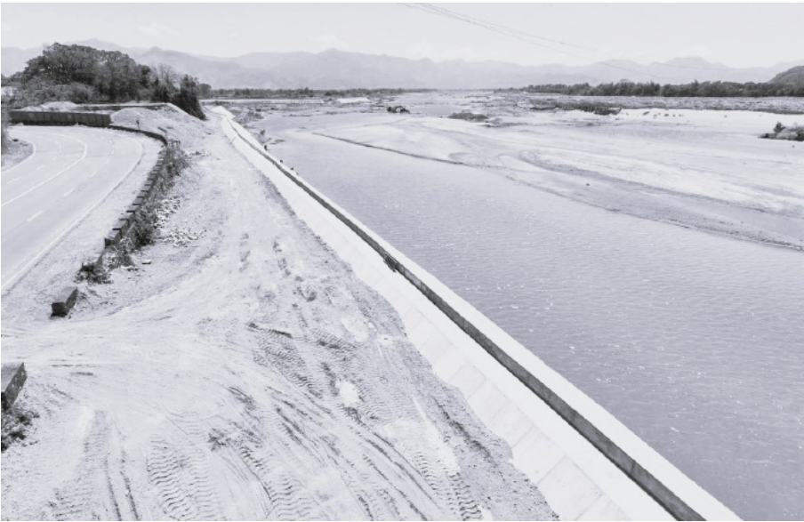
ties, and livelihoods from flooding especially as we prepare for the rainy season,” said Director Tan. Source: DPWH
